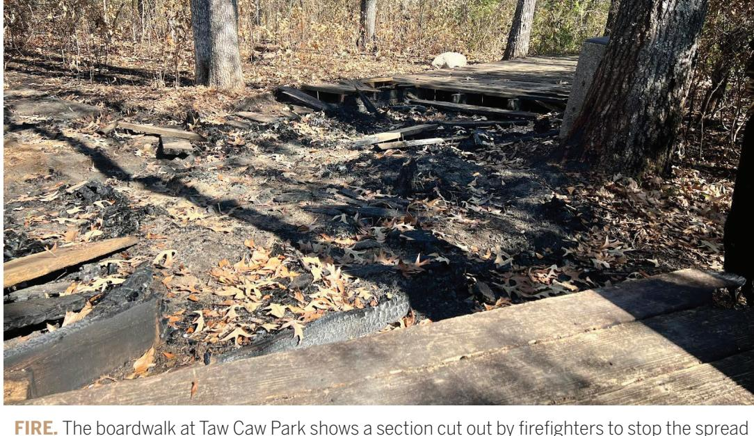
**FIRE.** The boardwalk at Taw Caw Park shows a section cut out by firefighters to stop the spread of flames after a Dec. 23 fire caused extensive damage to the structure. (Photo C/O Melissa Foust-McCoy)
