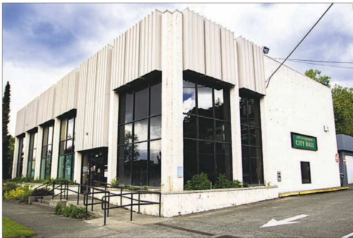
Chehalis City Hall is pictured in this photo captured last week.
