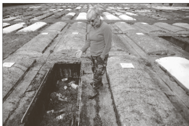
Jennifer Duncan, a former caretaker at Greenwood Memorial Park, shows trash in an open concrete burial plot on at the Centralia cemetery in April 2014. She was arrested for violating a restraining order by being at the cemetery Thursday.
