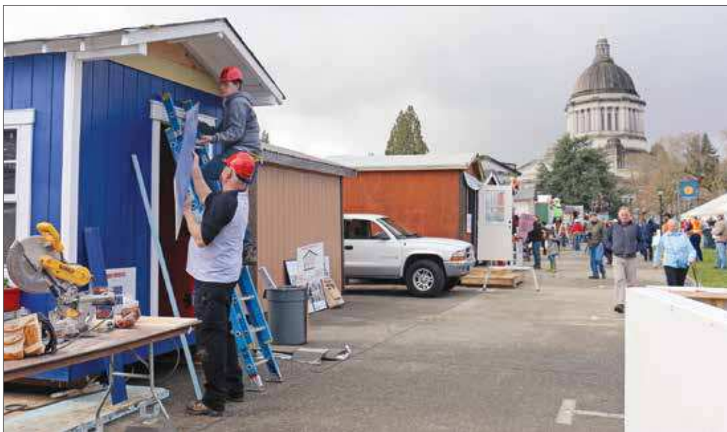
Students from Tenino High School add siding to their homeless shelter on Monday in Olympia.
