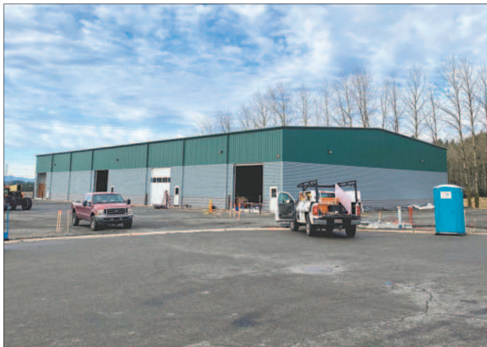
Port of Chehalis / Courtesy Photo The Port of Chehalis is inviting the public to a ribbon-cutting ceremony for the recently completed McBride Court Project.
